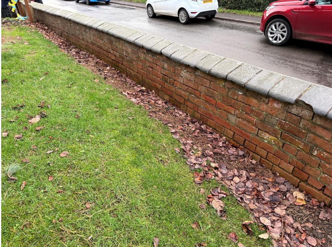
Image 3 – Image of rear of wall showing reduction in levels
