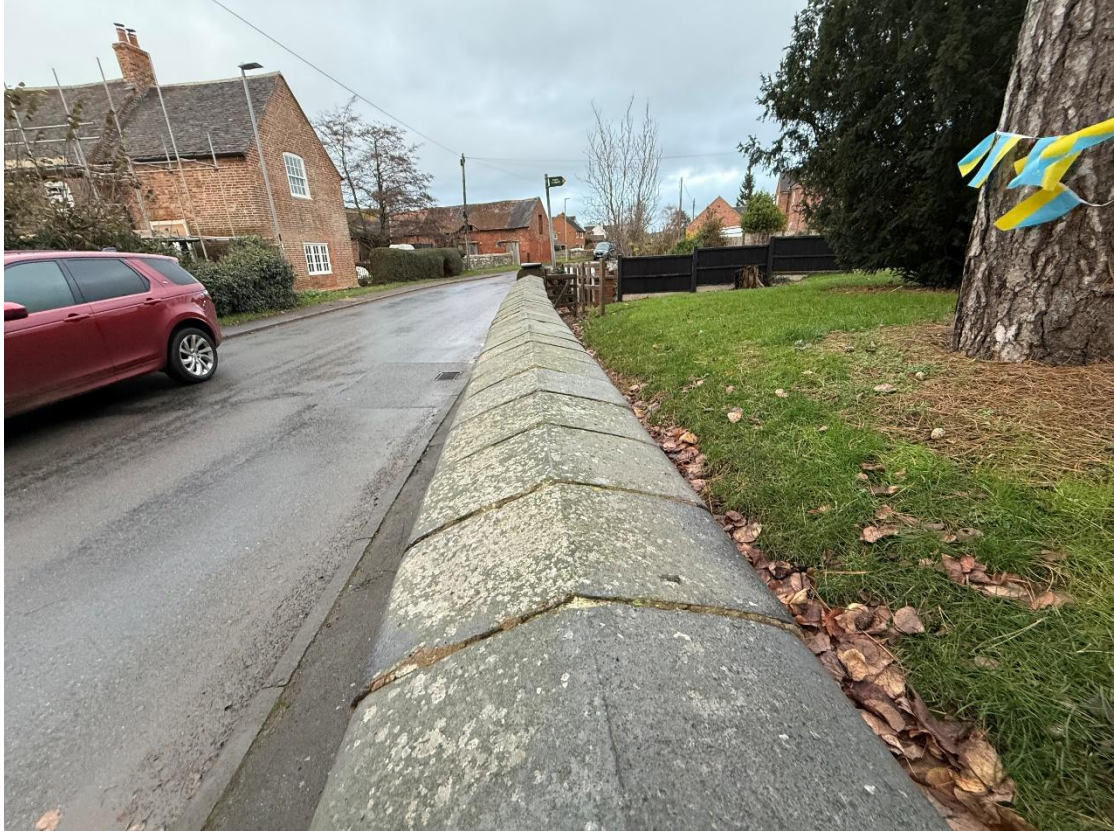
Image 5 – Image showing deviation in wall line
