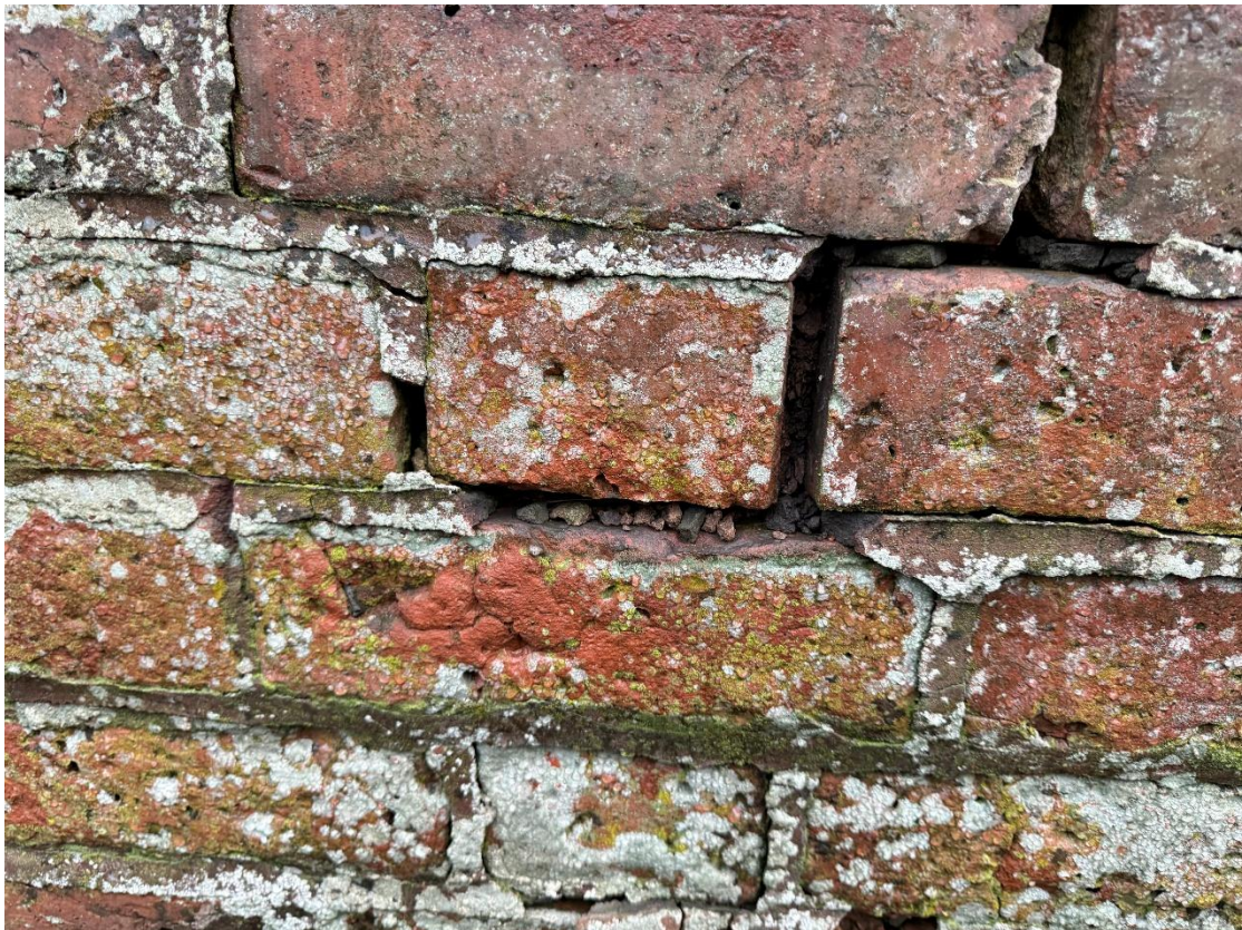
Image 6 – Image showing severe mortar loss
